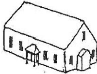
1891 #28 Converted to Community Centre
